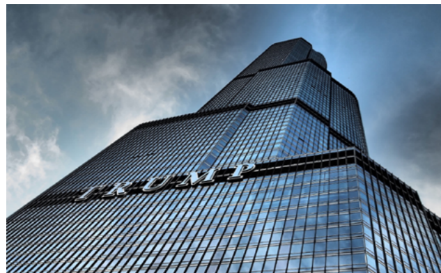
Der „Trump International Hotel and Tower“ in Chicago.
